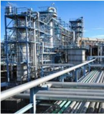
Power, Oil & Gas 電力石化油氣
